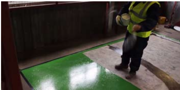
Provide sand powder for anti-skid need.
