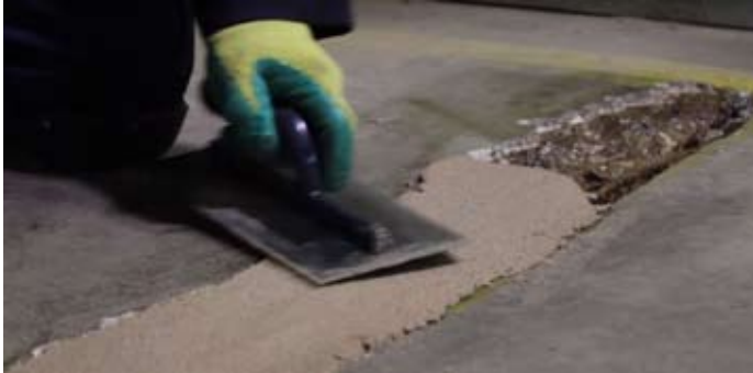
Grouting uneven area or big damage area.
