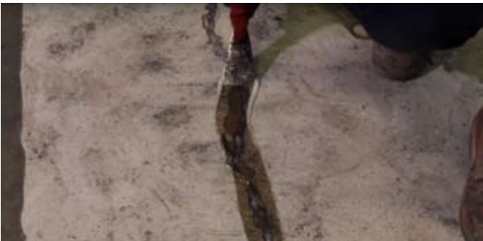
Patching cracking line by E-501S (+snad)
