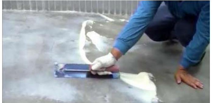
Provide putty filler E-501S or Provide Epoxy motar by E-501 + 6x~12x sand.
