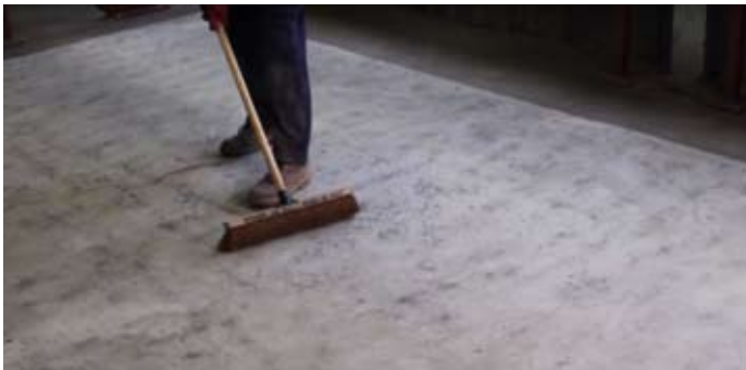
Sweeping and cleaning the surface free from dirt / dust.
