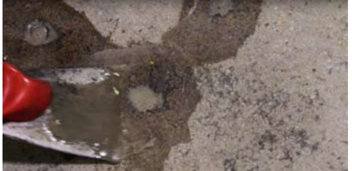
Hole patching by E-501S (+ sand)
